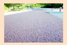
**Premix Seal Coat:** Premix is a mixture of fine aggregate, Portland cement filler, bitumen emulsions and additional water. They may be used to seal wide cracks, fill
