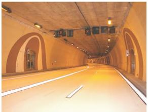
**BITUCLAIR** is a synthetic binder that remains translucent when applied in thin layers and takes on a honey-colored tint in thicker layers. It is manufactured with base products that do not contain asphaltene, the molecule that makes conventional bitumen black.
